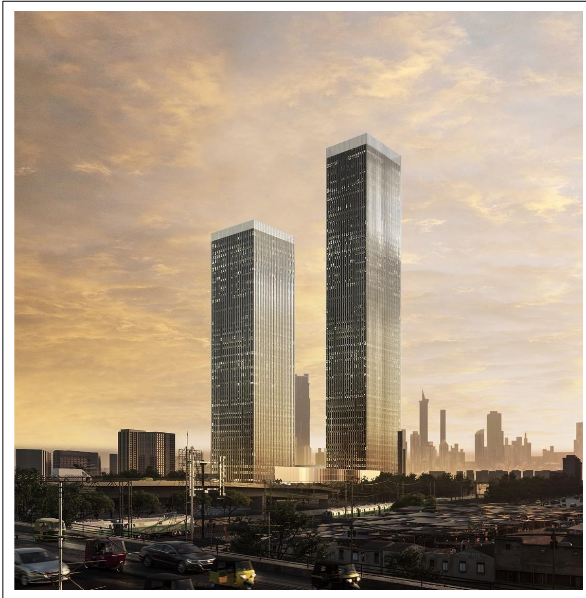
Prestige Liberty Towers, Prestige Group, Mumbai
